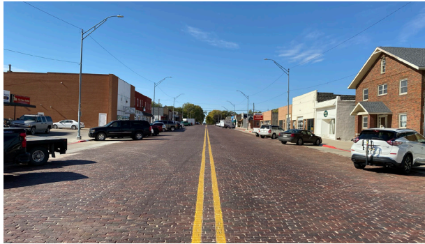
FIGURE 2.27 / BRICK SURFACING ON 1ST STREET DRIVE LANES
