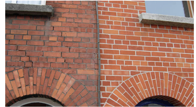
FIGURE 4.24 / BEFORE AND AFTER TUCKPOINTING MASONRY
