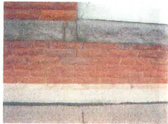
Window Stone Sill at North Exterior Wall
