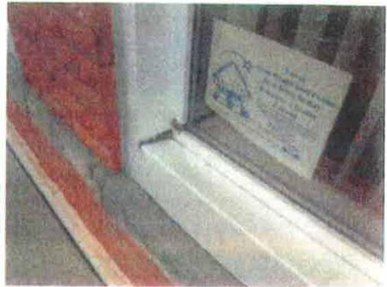
Window at North Exterior Wall
